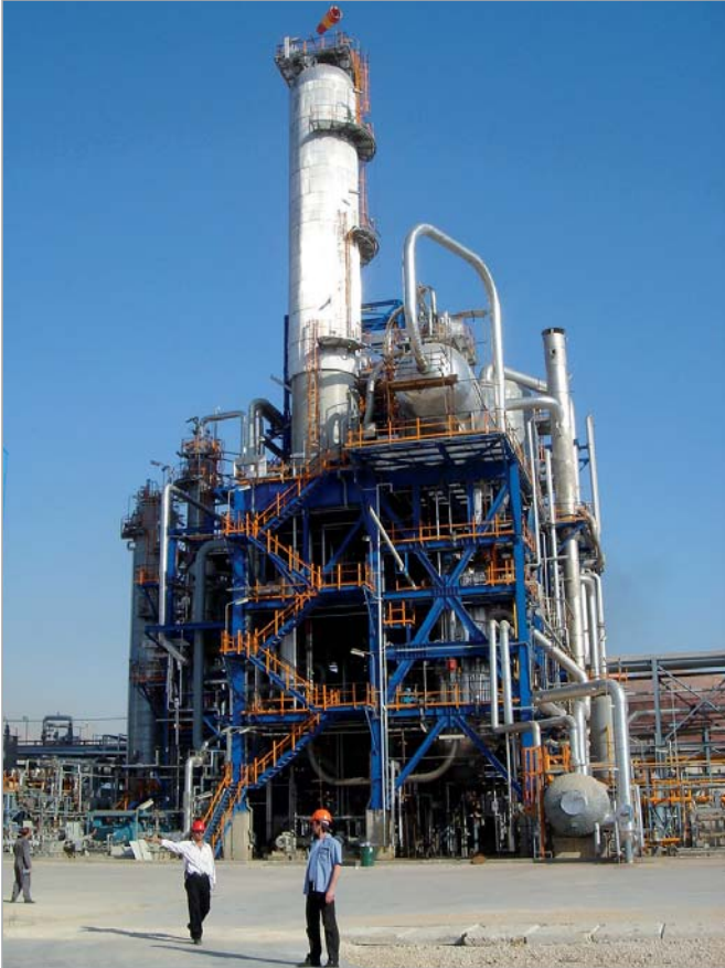
Stamicarbon Urea Plant
